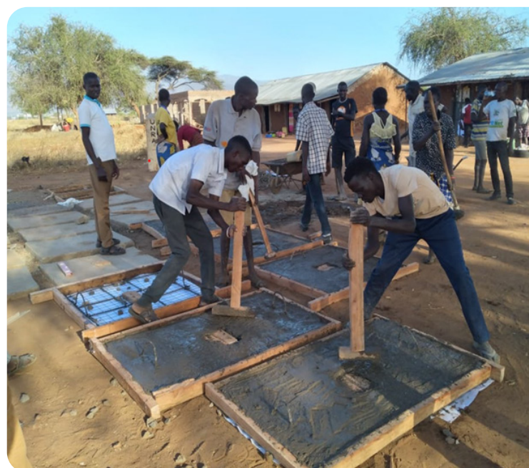
Entrepreneurs learn how to create concrete latrine slabs during training.
