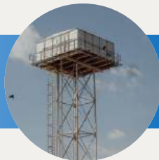
County Government and the USAID IPs supported installation of water kiosks at Bubisa community
